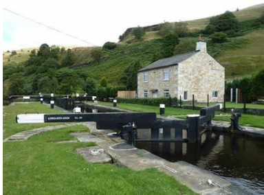
12 Lock / Lock gate signage
