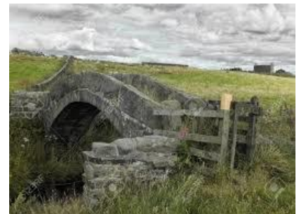
21 Old stone humpback style bridge
